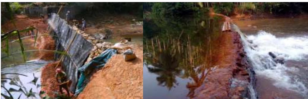
Fig. 27: (left) an underconstruction katta and (right) fully functional katta Source: https://www.deccanherald.com/
