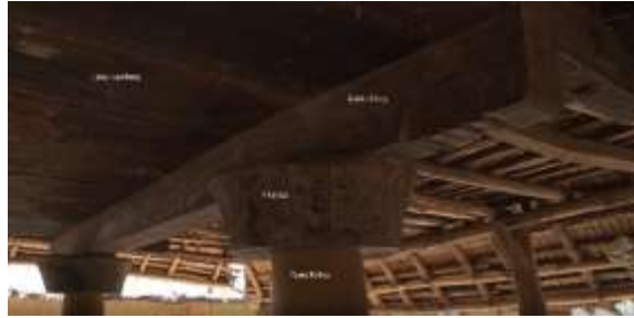
Fig. 6: View under the barn floor
