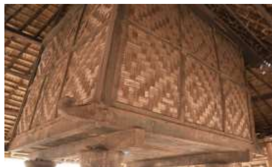
Fig. 5: The barn structure of Geleng
