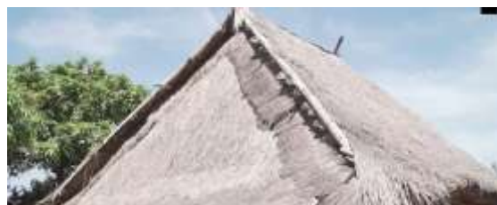
Fig. 7: The roof covering made of dried thatch leaves
