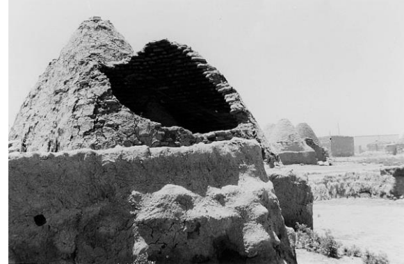
Fig. 7: A half ruined dome displaying the structure Source: Ozdeniz et.al, 1998
