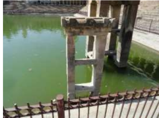
Fig 24: Traditional water control system constructed in stone - Thobu/Thoombu to regulate the flow of water out of the Panchakalyani into lower tanks
