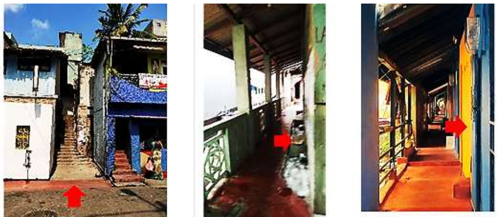
Fig. 4: Entrance stairways from the road to upper-level passage.
