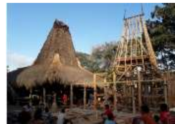
c. House Construction Process (August 2019)
