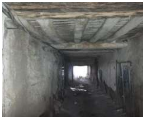
Fig.16: Current state of the covered alleyways. Source: Authors
