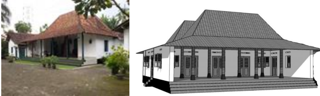
Fig 5: Transformation of House no. 7. Source: Survey, 2017
