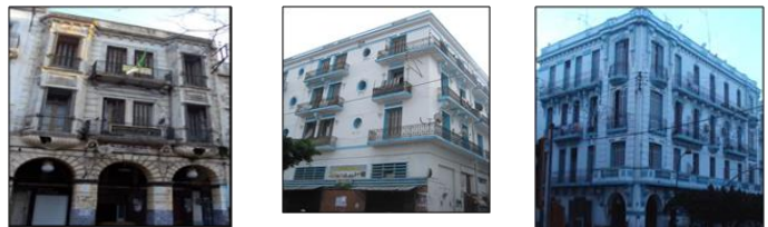
Fig. 3: Location and façades of buildings Source: author
