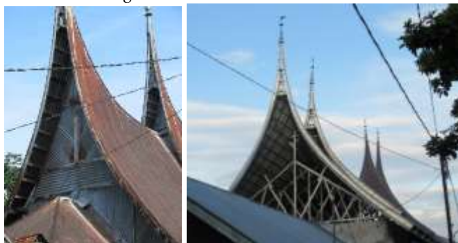
Fig. 3: Roof Metal Sheet Artistry of the 1980s and 2017 (3a ) The Use of Metal Sheet as New Craftsmanship, (3b) The Alien Authentic Rumah Bagonjong Style Source: author
