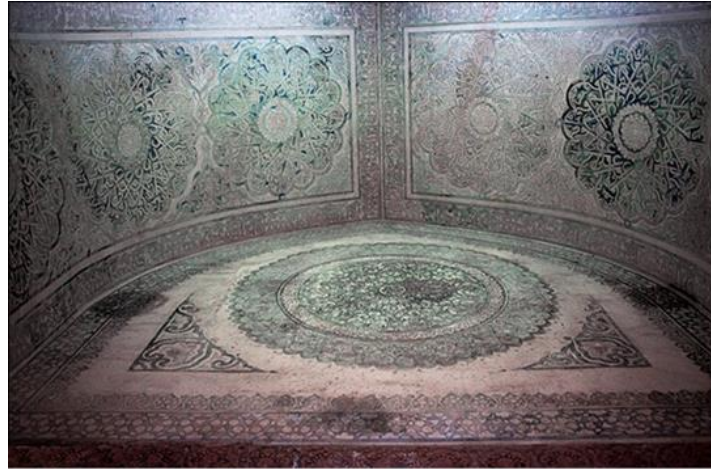
Fig 2: motifs of the roof interior view in Soltanieh Dome (Source: Author)
