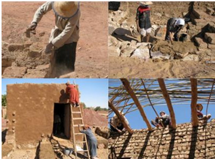
Fig. 8: The physical neo-desert vernacular model house during different work phases.
