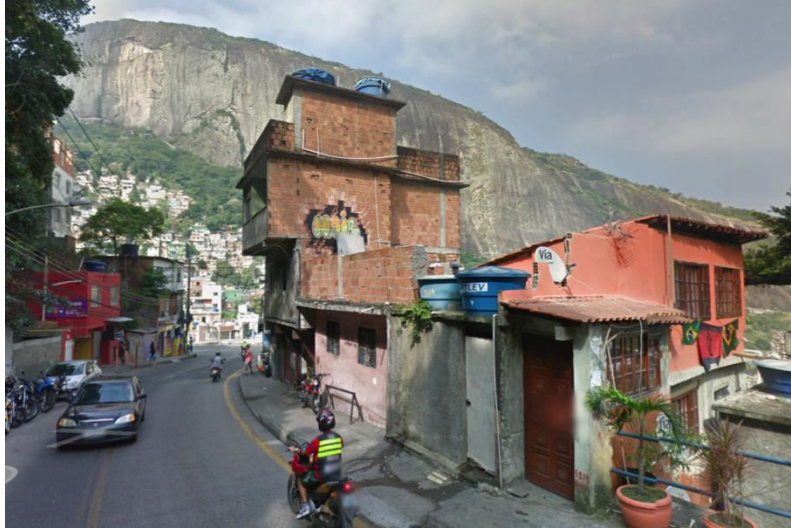
Fig. 10c. Construction type 3 in Rocinha. Massive overhangs are possible. 5 (Source: Google Streetview, May 2015)
