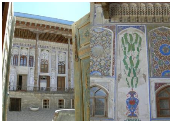
Fig. 13: Faizulla Khodjaev's house: iwan and decoration.
