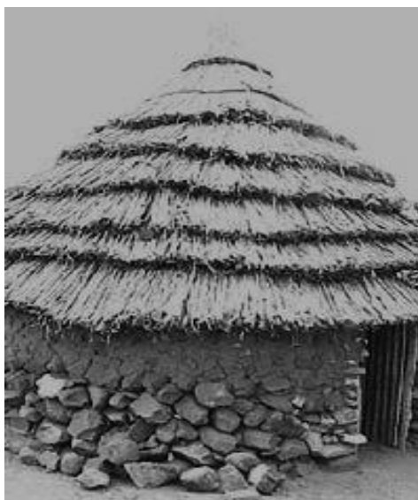
Fig. 9: An example of IDP houses built of mud and thatch
