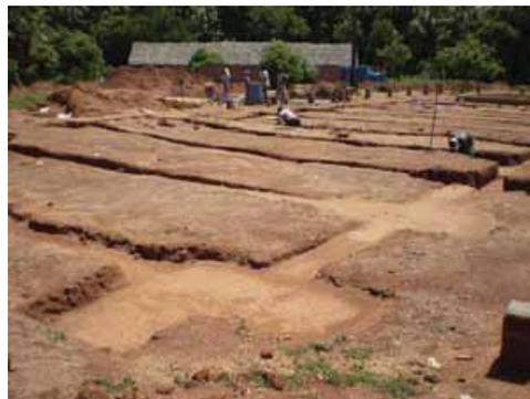
**Fig. 1:** Rammed Foundations
