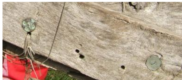
Fig. 12: Use of nails and coins for quick repair Source: Grainge, G.
