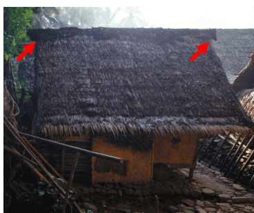
Fig. 13: A house in an outer Baduy village with slightly extended ridge (red arrow). Source: Kuncoro Widyo Rumpoko, 2013.
