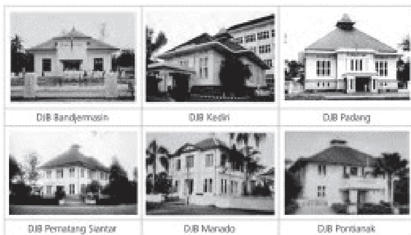
Fig. 9: De Java Bank Building in Indonesia
