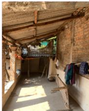
Fig. 11: Change of the wall materials, use of brick piers and asbestos roofs
