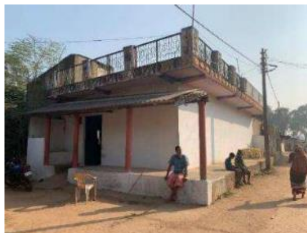
Fig. 13: Addition of a new structure
