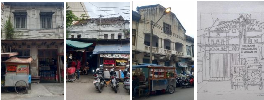
Fig. 8: Various Activities as Various Activities as a Lifeline for Empty Old Buildings around Pasar Baru through Photos and Sketch
