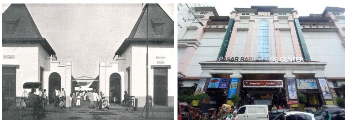
Fig. 1: The Façade of the Pasar Baru Building from the year of 1950 (left) & the year of 2022 (right).
