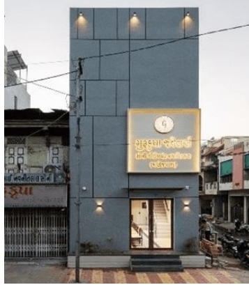
Fig. 14: Showroom Front Facade Source: Author
