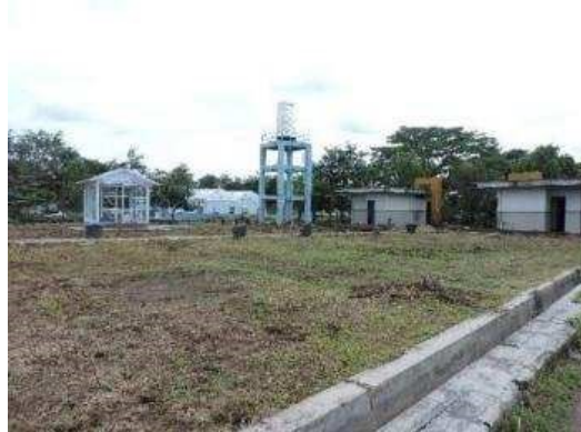
Fig. 12: Damaged Garden Area Source: Author, 2023
