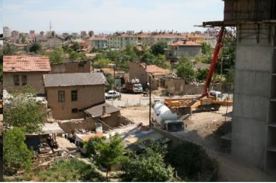
Fig. 9: Photo of Saim Sakaoğlu House neighborhood Source: Author (09.03.2009)
