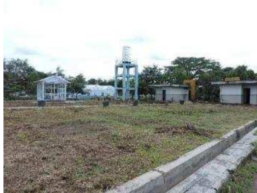
Fig. 12: Damaged Garden Area Source: Author, 2023
