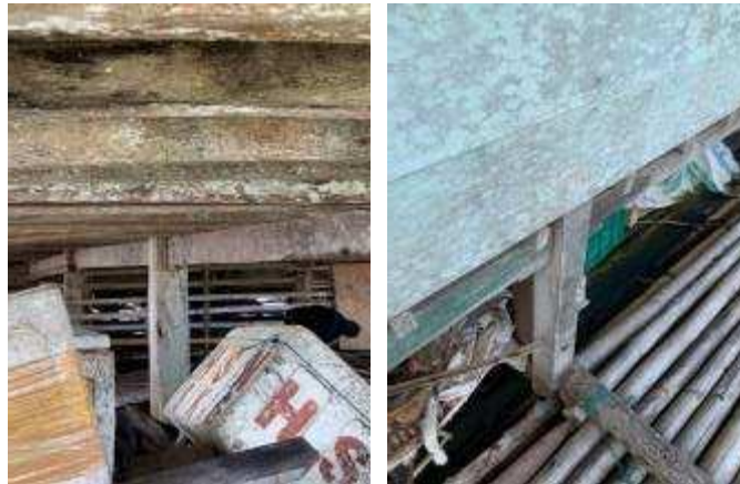
Fig. 8: Columns on a floating house Source: Author documentation, 2023
