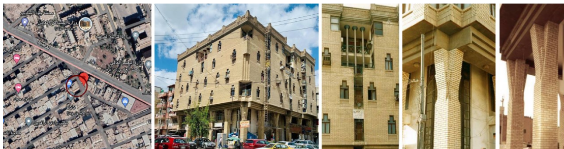
Fig. 5: Location and design of Building "Eya", Al-Bataween in Baghdad - Iraq Source: Al Chalabi, 2019.
