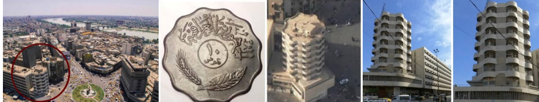
Fig. 4: Shows the location and design of The Department of Labor and Social Affairs building in Baghdad - Iraq Source: Al Chalabi, 2018.
