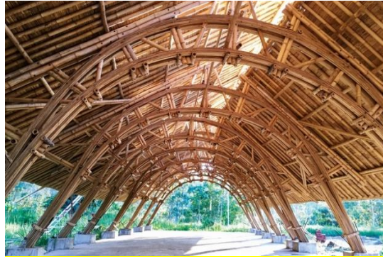
Fig. 7: Trusses/ roof Source: Yadav, 2021
