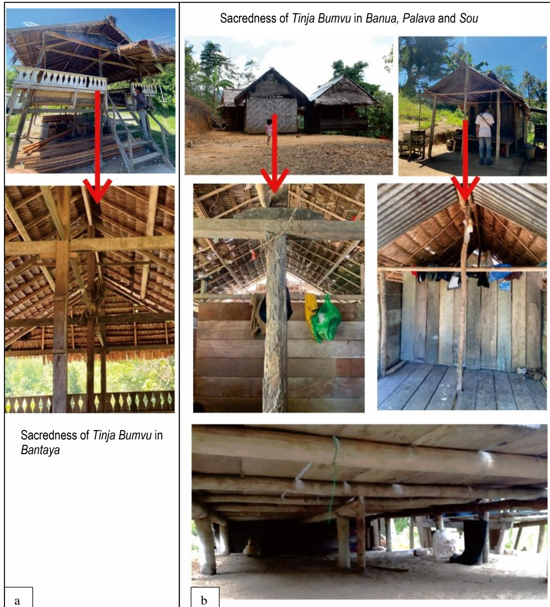
Fig 4: TinjaBumvu (king's pillar), in (a) Bantaya and (b) Sou that continue to Soil.
