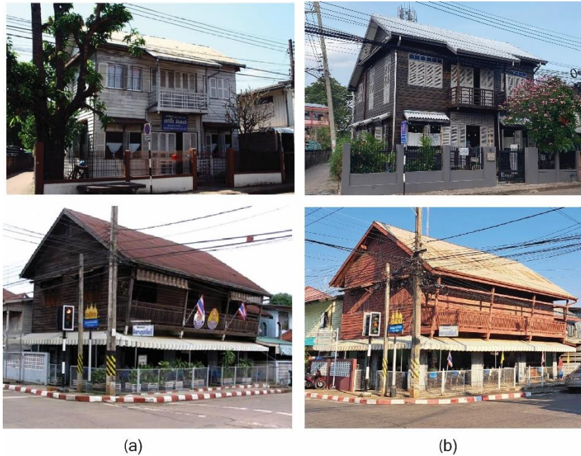
Fig. 9: (a) vernacular row houses before renovation in 2007 and (b) the vernacular row houses after renovation by building owners in 2022.
