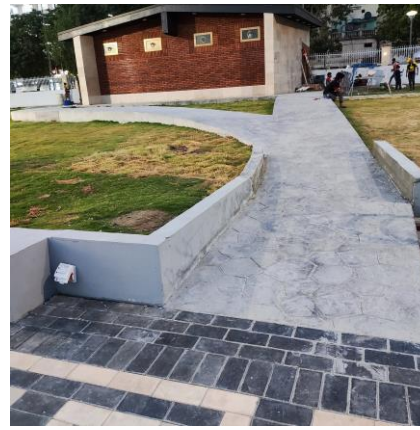
Fig. 17: The ramp to the WC.
