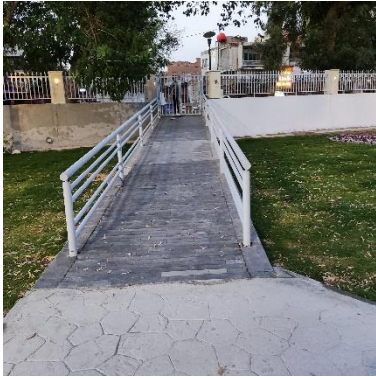
Fig. 13: Secondary entrance with ramp without tactile surface or construct warning strip
