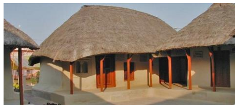
Fig. 4: Chala roof of Bengal in Vernacular Architecture. Source: Naveen Nishant, 2023
