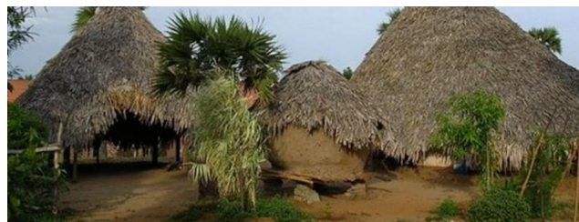
Fig. 9: Chutillu round house of Andhra Pradesh can withstand cyclone Source: Serene Sarah Zachariah (thebetterindia.com).
