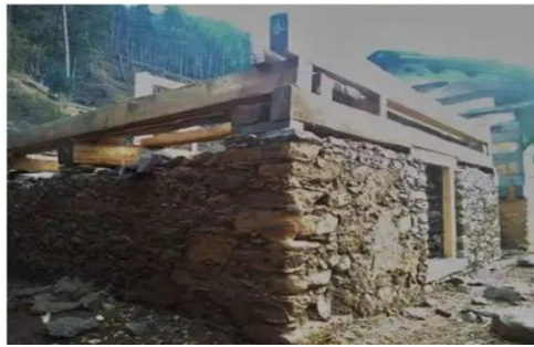
Fig. 3: Koti Banal Construction process (Uttarakhand) Source: Saraswat, 2017.
