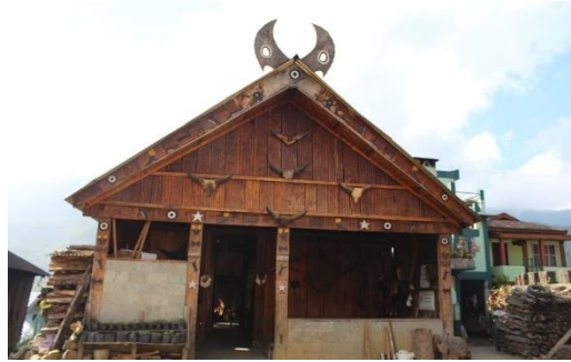
Fig. 2: Morunga youth dormitory of Konyak Naga (Nagaland) Source: Praween Kumar, 2020
