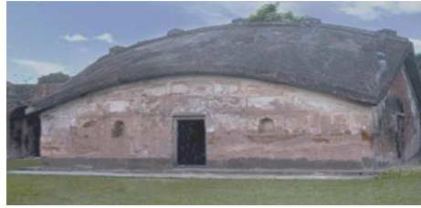
Fig. 2: Chala roof in rigid material at Fatah Khan Tomb, Gaur, Malda, West Bengal, India. Source: Naveen Nishant, 2023
