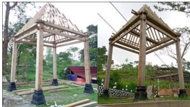
Fig 1: Structure System of a Joglo Traditional Building.
