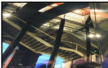
Fig. 12 : The vertical movement system in the building, and the modern finishing materials used.
