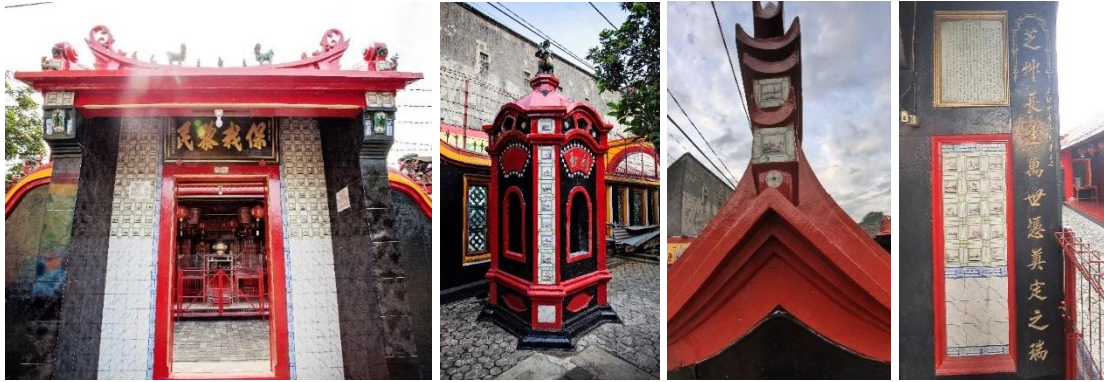
Fig. 8: Ceramics on the entrance walls, kilns, roofs, and walls in the temple
