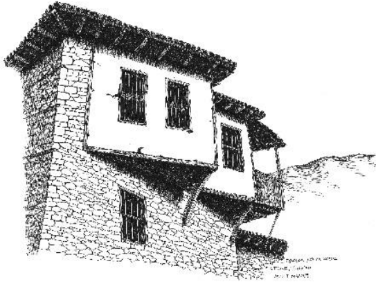
Fig. 3a: Jetty, rural house, Stence, Tetovo region
