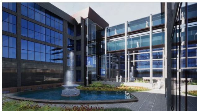
Fig.7: The central courtyard to provide natural lighting and ventilation for the spaces overlooking it. Source: Al-Bajari/ the Department of Architecture, University of Technology.
