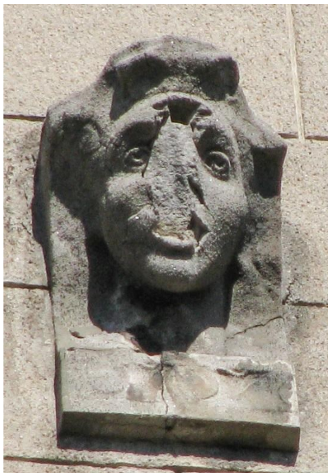
Fig. 12. Damaged mascaron, 20-22 acad. Hnatiuk Str., arch. R. Felinskyi, with the participation of F. Kessler, sc. Z. Kurchynskyi, 1910 Source: created by the author.
