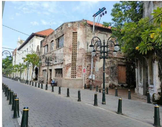
Fig. 17: Unmaintained buildings Source: Author, 2022
