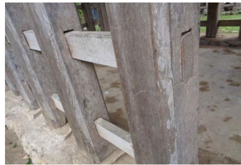
Fig. 9: Detail for Tongkonan pile joint: (a) Using the pedestal foundation; (b) Post connection system Source: Author
