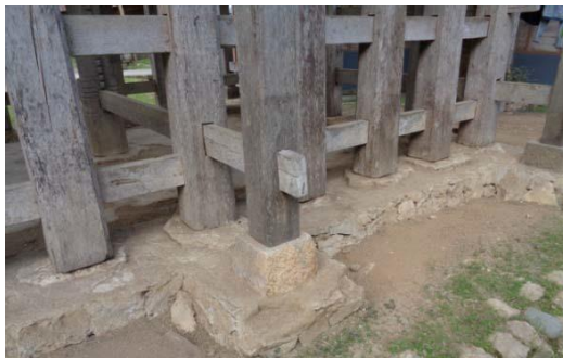
Fig. 9: Detail for Tongkonan pile joint: (a) Using the pedestal foundation; (b) Post connection system Source: Author
