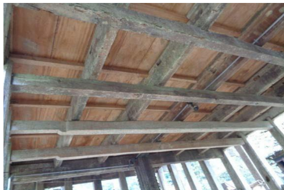
Fig. 10: Tongkonan beam construction Source: Author
