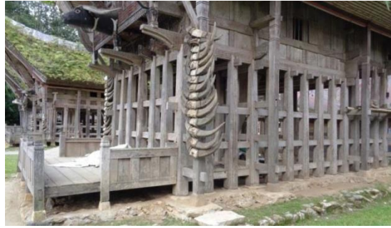
Fig. 8: Tongkonan pile construction Source: author
