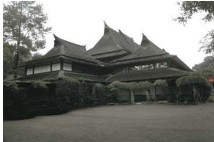
Fig. 1: The East Hall of the Bandung Institute of Technology Source: Author, 2023
