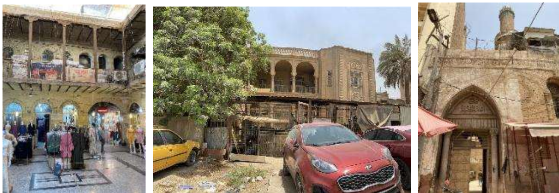
Fig. 4: Historic buildings on Al Nahar Street A. Khan AlKhudairi, B. Al-Adelia Mosque, C. Building at the riverside. B. Source: Authors
