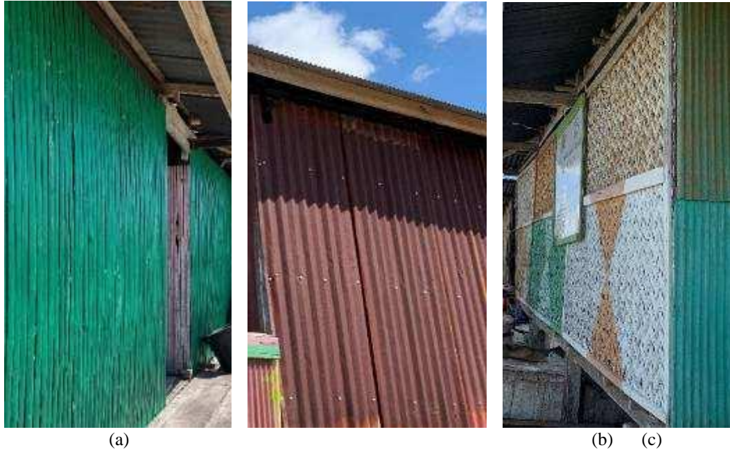
Fig. 20: (a) Walls made of split bamboo (salima), (b) Walls made of zinc, (c) Walls made of woven bamboo
