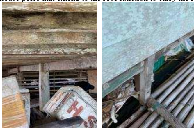
Fig. 8: Columns on a floating house Source: Author documentation, 2023
