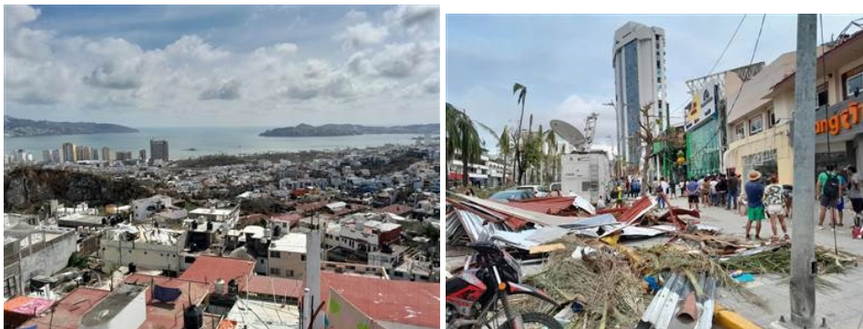
Fig. 4: Acapulco, devastation after the hurricane. Source: Author, 2023.
