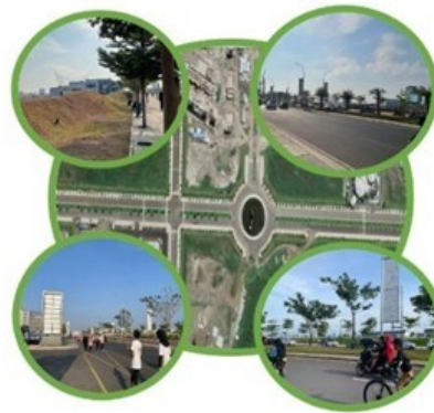
Fig. 5: The condition along CPI road area
