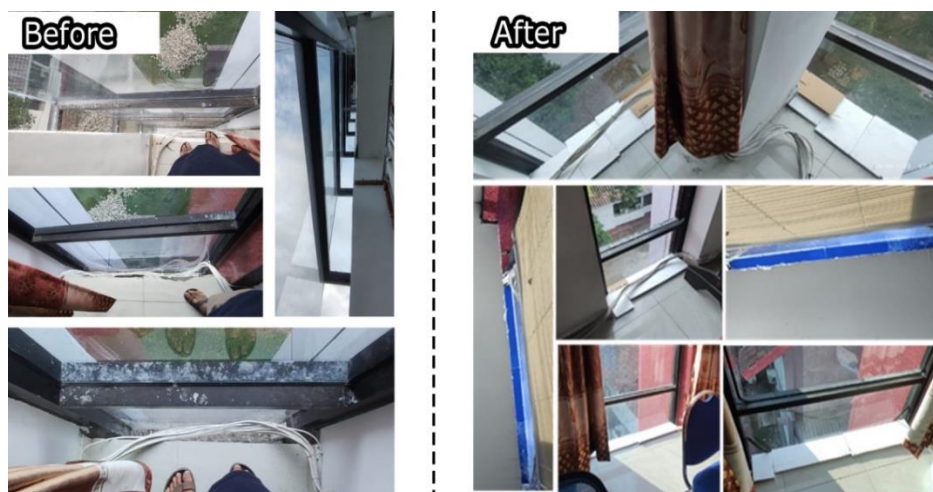
Fig. 5: the office room situation by closing room gaps using cork styrofoam.
