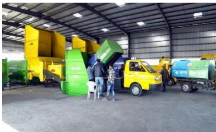
Fig 9: Garbage Transfer Station
