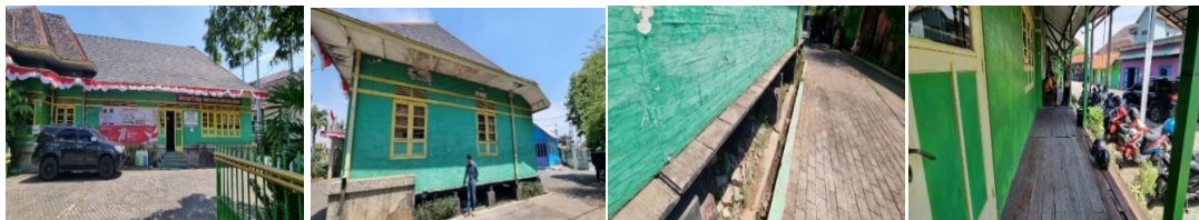
Fig. 8: The building by the Dutch East Indies government. It used to function as a Bumiputra school. The stilt building, the walls and floors are made of wood.
