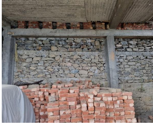
Fig. 10: Stone wall with RCC columns, slabs and concrete band Source: Author
