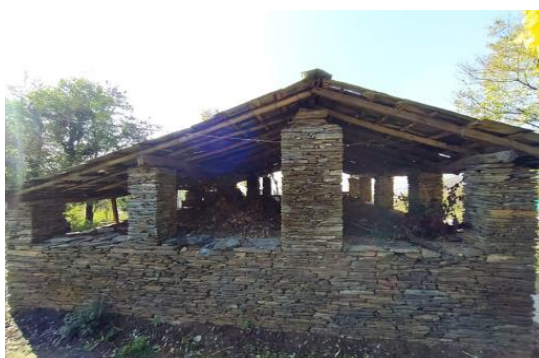
Fig. 4: A House with Dry Stone Construction Source: Author
