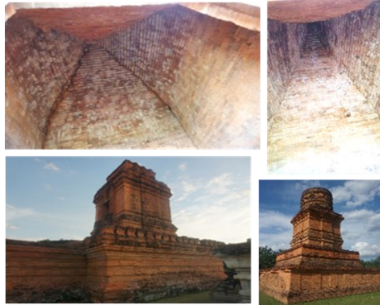
Fig. 10: Brick Temple in North Sumatra using the terraced corbel such as Si Pamutung and Bahal Temple
