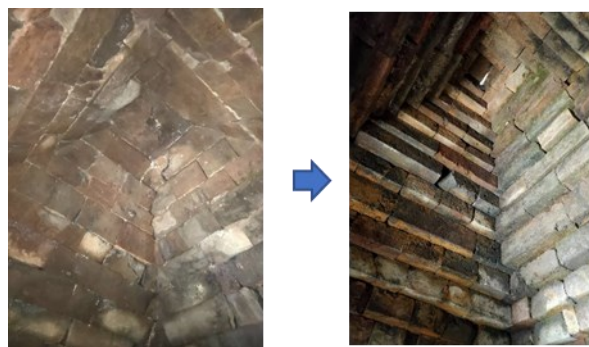
Fig. 6: The Ceiling Development in Dieng Temple Source: Rodriguez, 2020
