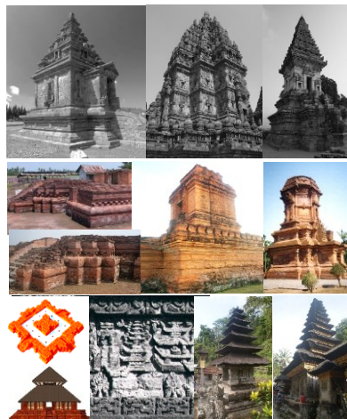
Fig 1: Early Classical Era (4-7 AD) (left), the Middle Classical Era (8-12 AD) (middle) , and the Late Classical Era (13-16 AD) (right). Temple materials in Indonesia: Stone (Upper), Brick (middle), A picture of a wooden building and its combination with brick or stone (below) Source: Herwindo, 2022
