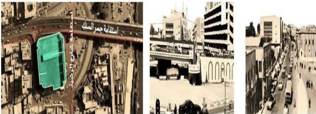
Fig. 4: The straightness of the Al-Sinak bridge before and after its construction
